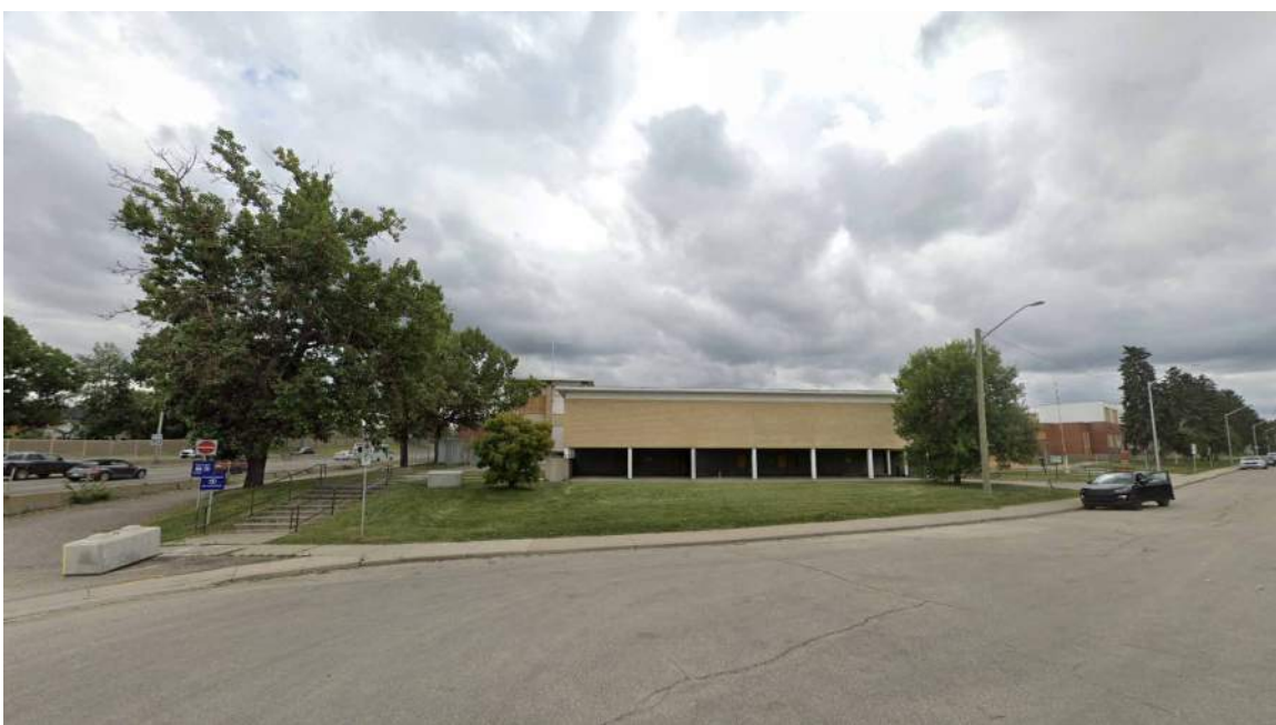
B - SITE PHOTOGRAPH - NORTH EAST CORNER
